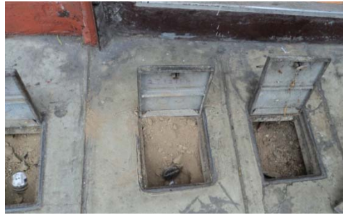
Figure 11 - Status of some water meter boxes
