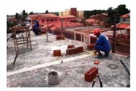
Figure 11: Marking the masonry
