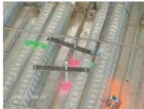
Figure 2: Color coding shows locations for sheet metal straps and pipe hangers on metal decking
