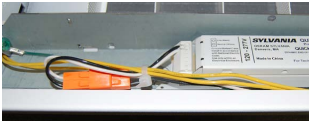
Figure 5: Wiring plug for ballast inside light fixture (Source: Picture by Iris D. Tommelein taken at Finelite, Union City, CA, 2008)
