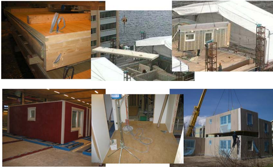
Figure 2: Illustration of the element and volume production system (Björnfort and Sardén 2006)
