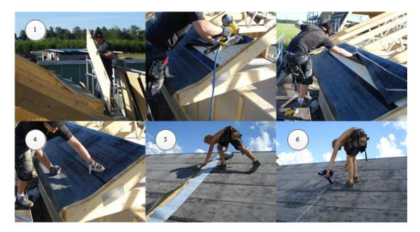
Figure 4: On-site assembly of product B
