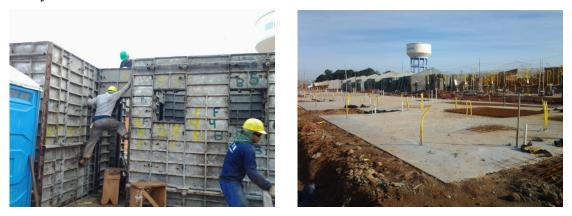
Figure 7: – Examples of improvisation: worker supporting himself on the concrete wall formwork (left) and inadequate electricity pipes in the raft foundations (right)
