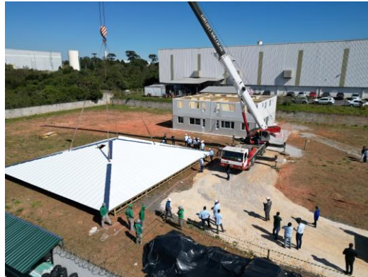
Figure 4: Two-Story Prototype built off-site.
