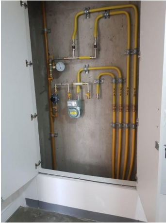
Figure 5: Pressure test
