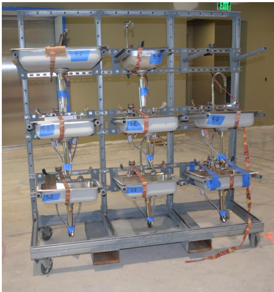
Figure 4: Example of lean logistics - cart with pre-assembled fixtures (Source: I. D. Tommelein, 20 April 2016)
