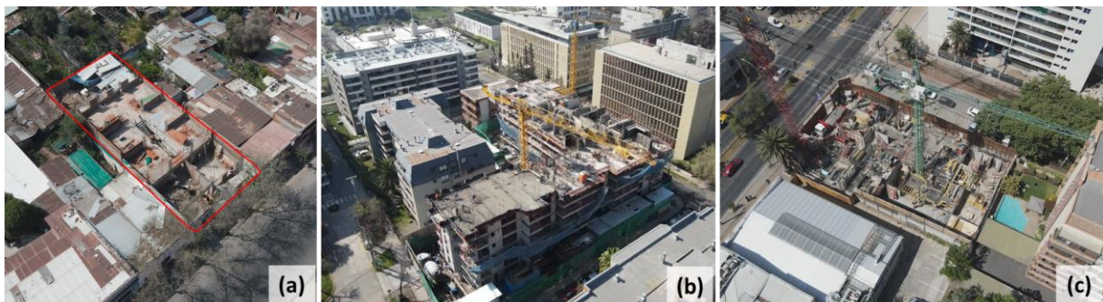
Figure 1: Case Studies: (a) 2-story reinforced concrete and confined masonry building (384 m 2 ); (b) 7-story reinforced concrete building (approx. 2,000 m 2 ); (c) 7-story reinforced concrete building (approx. 900 m 2 ).
