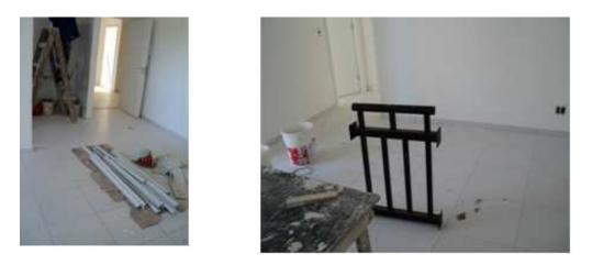
Figure 4: Improper storage of materials
